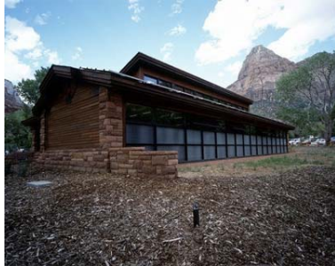
Zion's Visitor Center showing thermal storage wall and clerestory windows
